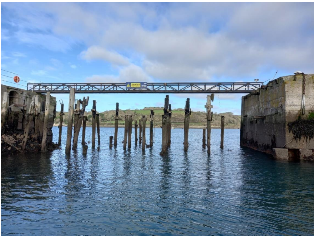
Figure 2-4: Timber Piles and Gang Walkway adjacent to the Northern Arm, looking north, Ramboll image 2022
