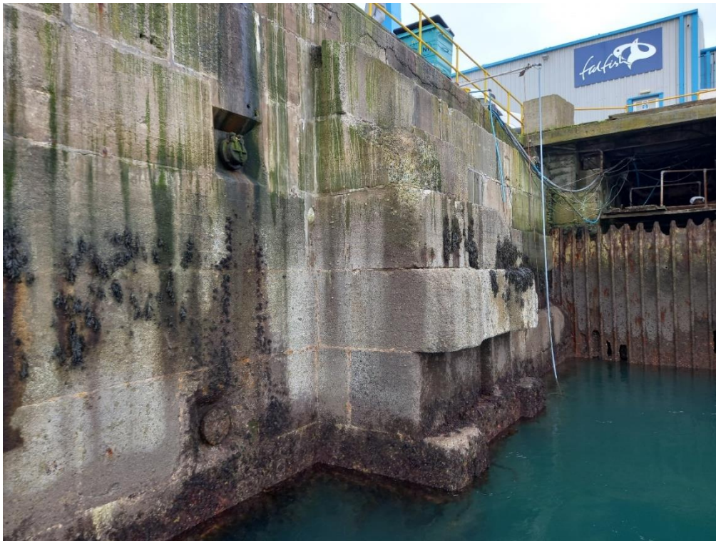
Figure 2-7: FalFish Site at the southern end of the Western Wharf, looking west, Ramboll image 2022
