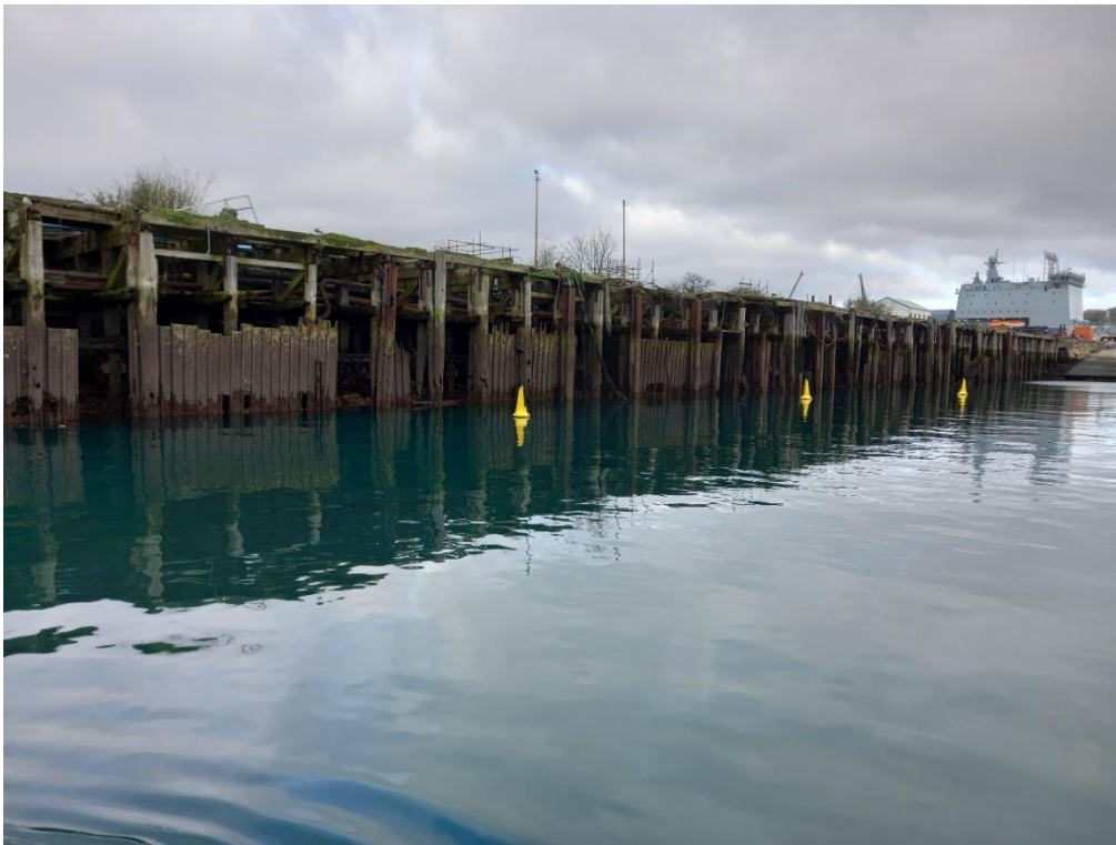
Figure 2-5: Western Wharf, looking northwest, Ramboll image 2022
